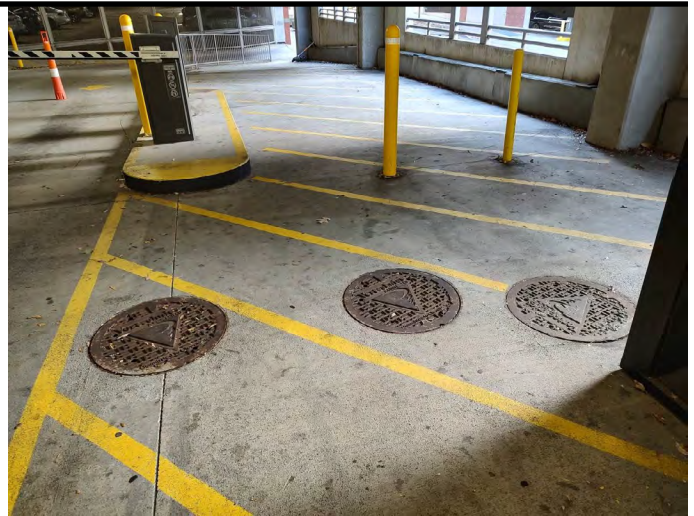
Market Square Parking garage sediment trap and oil interceptor covers (Downtown, Knoxville, TN)
