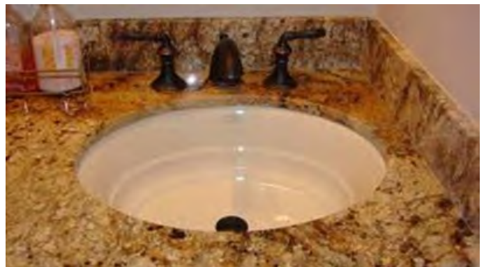
Under counter lavatory with projecting rim, 8” on center hole faucet and short lever handles
