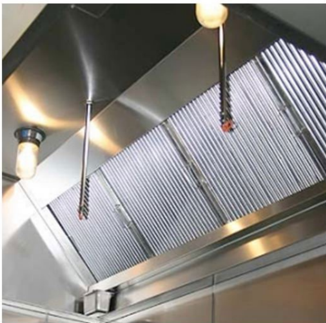
Commercial hood enclosure, filters, lights, and fire suppression nozzles
