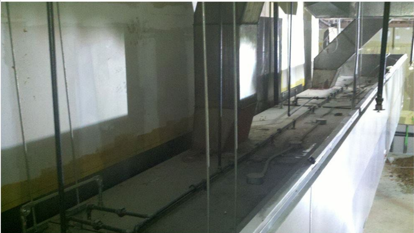
Range hood welded exhaust duct
