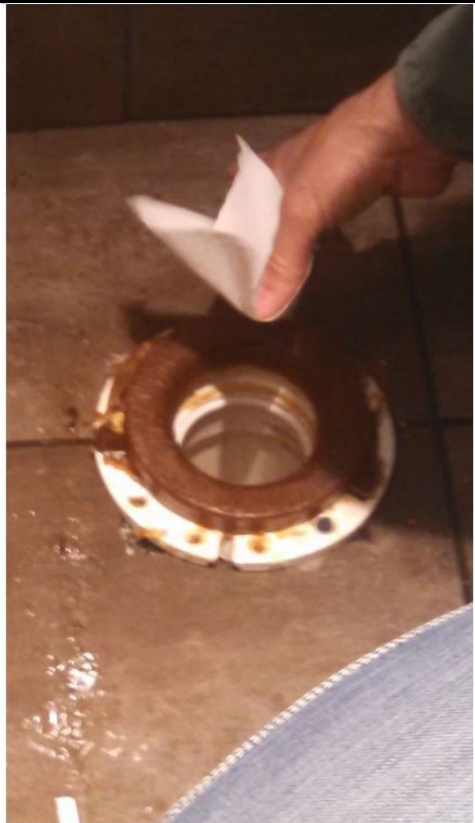
Toilet paper being blown upwards from airflow into restroom from the range hood exhaust fan
