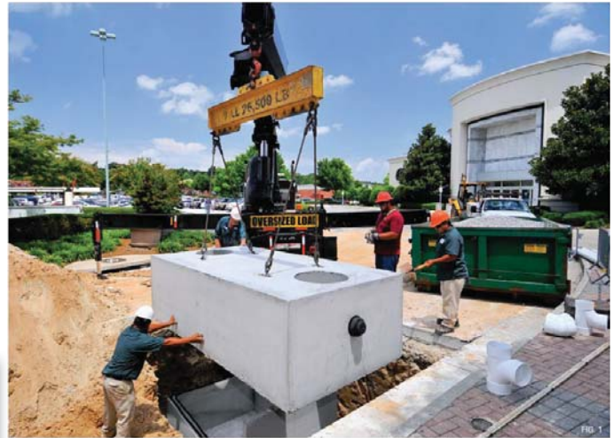
Exterior concrete grease interceptor installation
