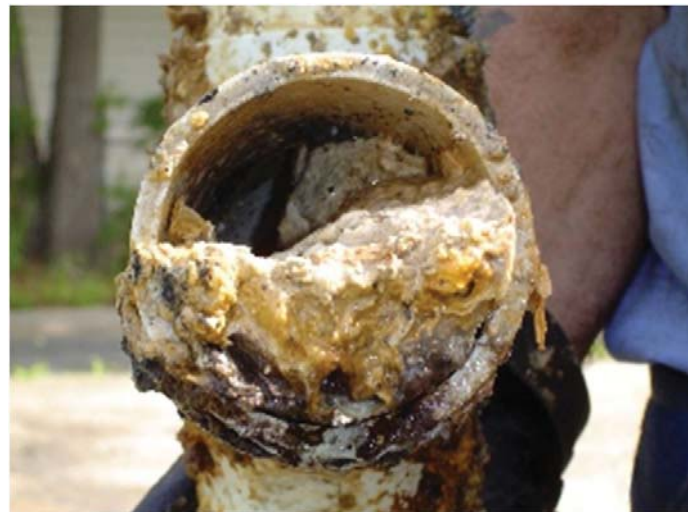
Grease clogged sewer line
