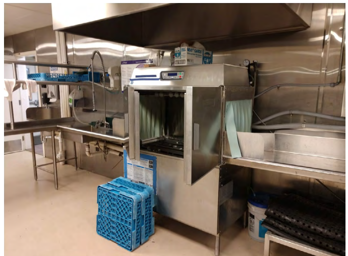
Dishwasher with large condensate removal hood
