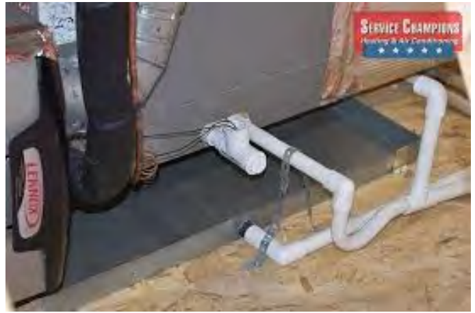
https://servicechampions.com/how-does-condensate-drain-pan-work/ HVAC unit condensate drain line
