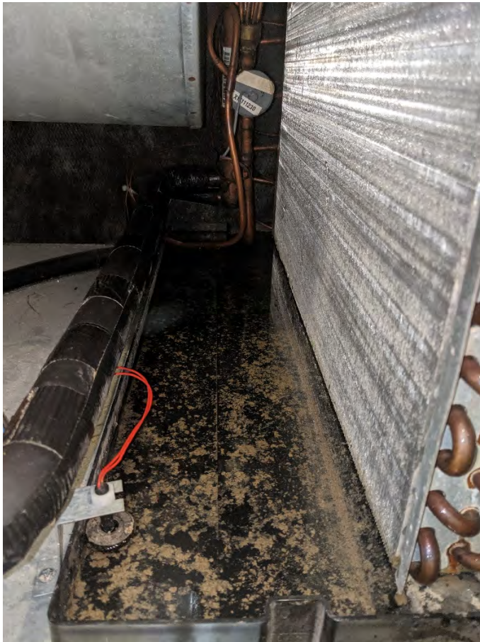
https://hvacbeginners.com/air-conditioning-condensate-drain-line-clogged/ HVAC unit condensate drain pan full of debris
