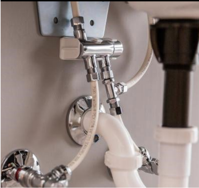
POINT OF USE MIXING VALVE UNDER LAVATORY
