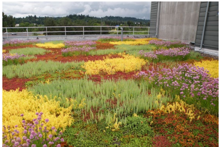
Installed vegetated roof assembly
