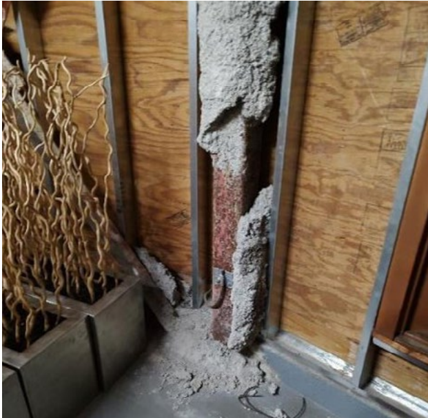
DAMAGED FIREPROOFING
